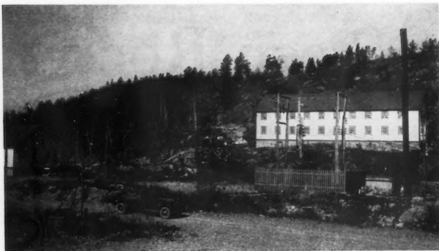
• • • Bunkhouse with capacity for 100 men. Secondary sub-station in foreground
